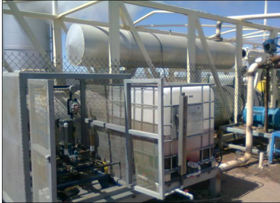
Figure 10. The Test Heat Exchanger
