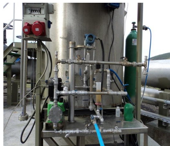
Figure 7: Photo of Inhibitor Dosing System
