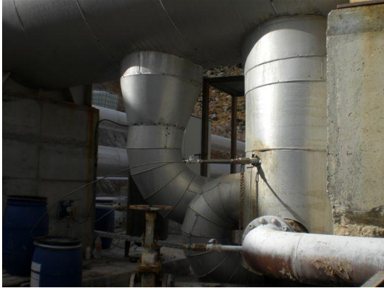
Figure 7: Photo of dosage point for iron dispersant.
