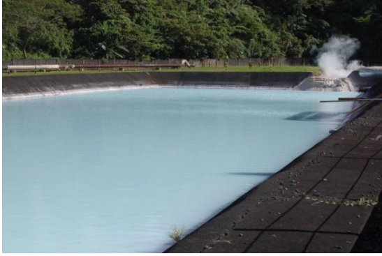
Figure 8 The sump riser has been eliminated from this sump and a low dam was built just upstream of the outlet.
