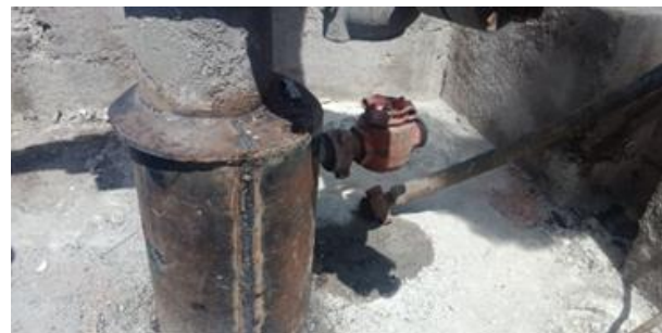
2. Welded casing ready for the squeeze operation
