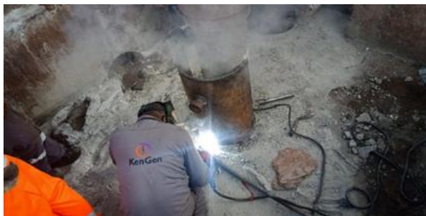
1. Welding the containing casing in place
