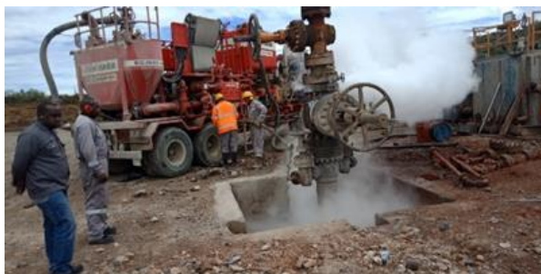
3. Conducting the cementing squeeze operation
