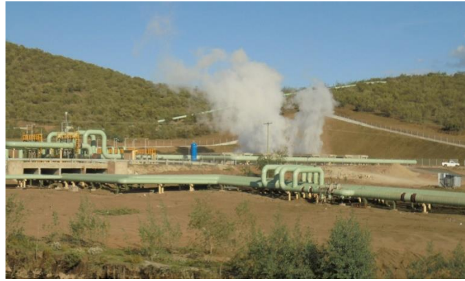
FIGURE 8: Olkaria IV separator station
