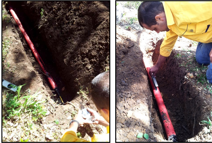
FIGURE 29: ICE technical staff placing, aligning and levelling the magnetic coils
