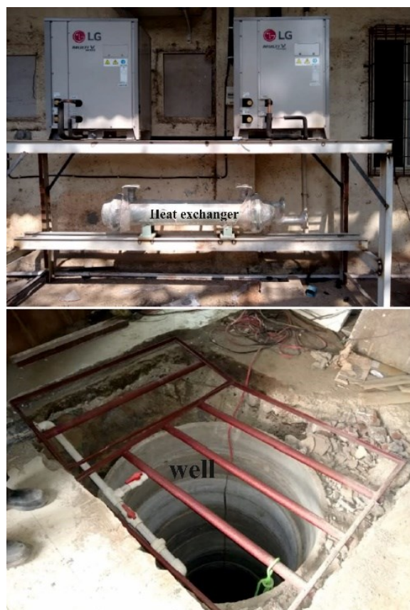
Figure 3: GHP unit installed in a pharmaceutical storage facility.
