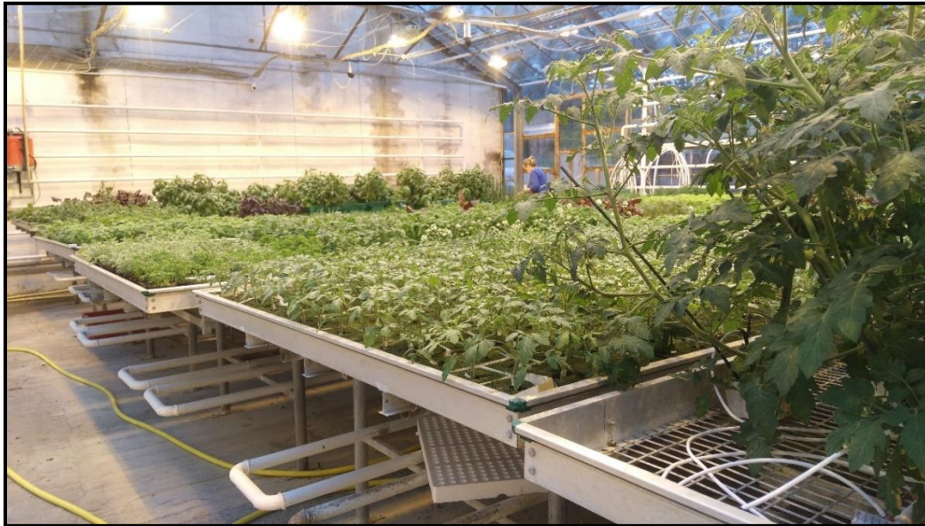
Figure 1.8: Heating pipes under the plant benches, on the side of walls in an Icelandic greenhouse.
