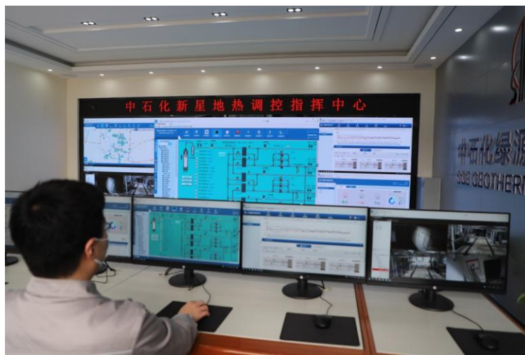
Figure 6: the IDH Control Center built by the JV in Xiongxian of Xiong'an New Area is connected with all subsidiaries' networks to realize remote monitoring.
