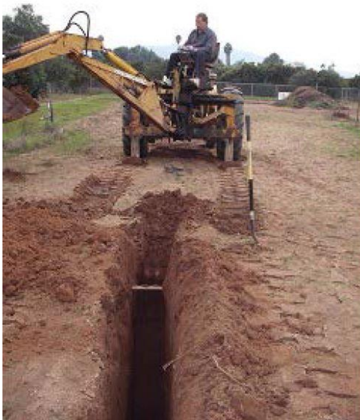
Figure 3. Land preparation for piping an EAHE
