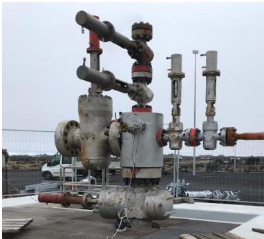
Figure 5: IDDP 2 arrangement of IDDP 2 wellhead
