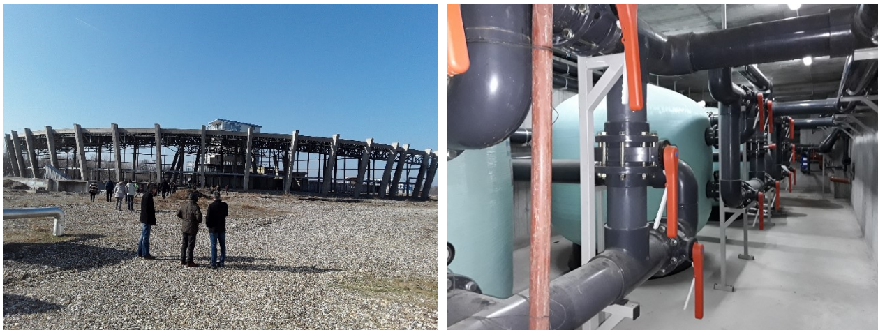
Photo 2. Slobomir - indoor swimming pool under construction (left) and subsurface installations for geothermal heating of the pool (right).
