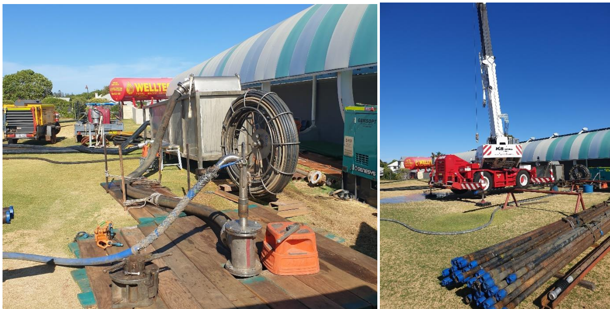
Figure 13. Example of rig-less workover to maintain injectivity of a 1 km deep geothermal system that has been operating for 12 years in Perth.
