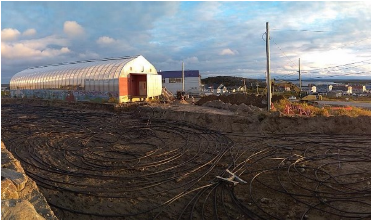
Figure 11. Kuujjuaq: Geothermal pilot project 30 kW horizontal GSHP system for Kuujjuaq, Quebec community swimming pool.
