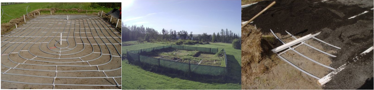
Figure 3: Piping layout (left), heated garden test bed at the Agricultural University of Iceland (middle), and in progress construction detail showing the pipes and the gravel drainage layer (right).
