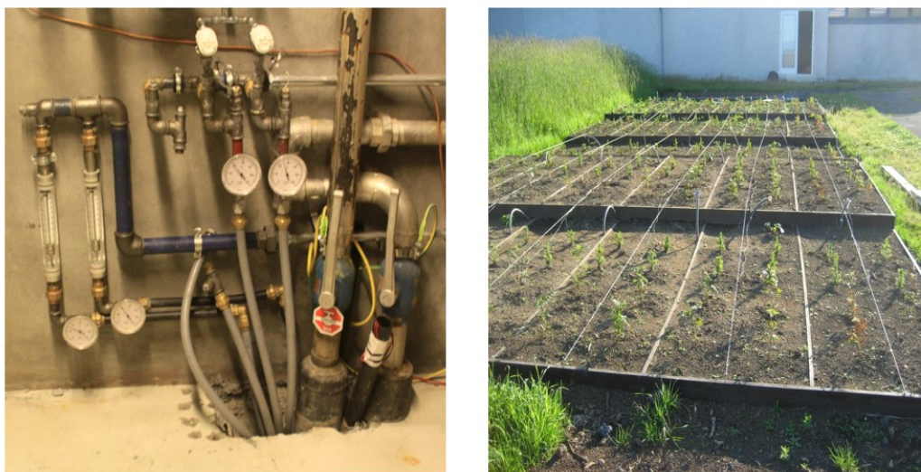
Figure 5: Keilir garden hot water distribution and monitoring system (left) and the finished heated garden (right).
