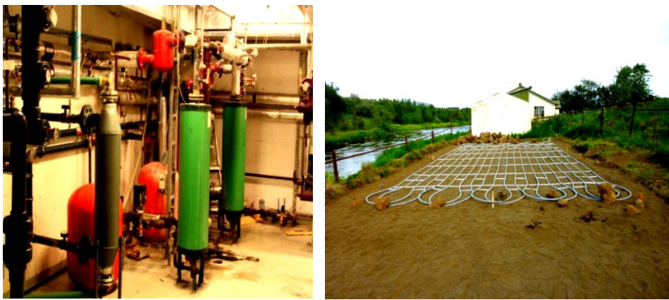
Figure 4: NLFI swimming pool heat exchangers (left) and the garden pipes before the gravel layer and the top layer of soil were added (right).
