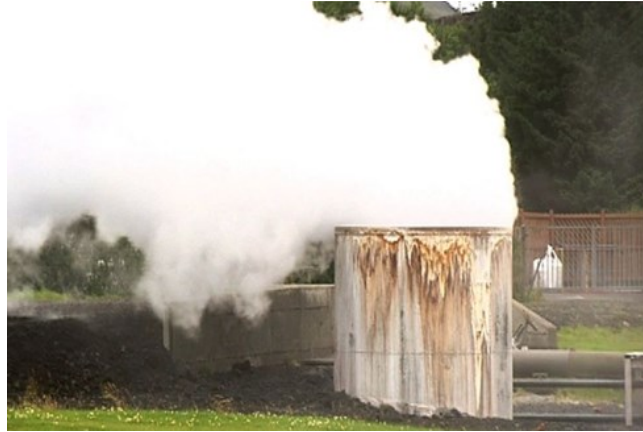
Figure 4: Geothermal steam from a silencer in Hveragerði (Veitur, 2018).
