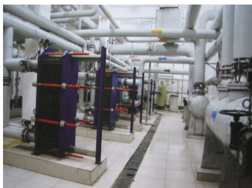
Figure 5 Geothermal Station with Indirect Heating
