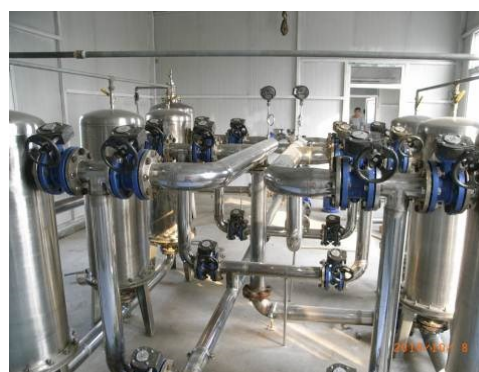
Figure6 Geothermal Recharge System
