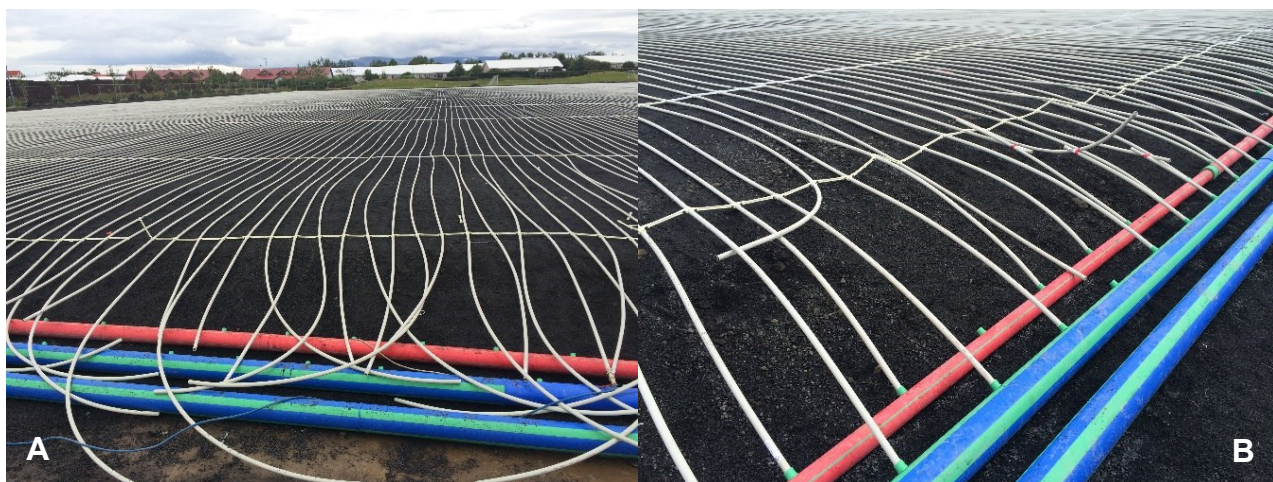
Figure 6: Lay-out of longitudinal loops with direct connection to the mains supply; a) Overview of the field; b) Detail photo at the connection to the mains supply.
