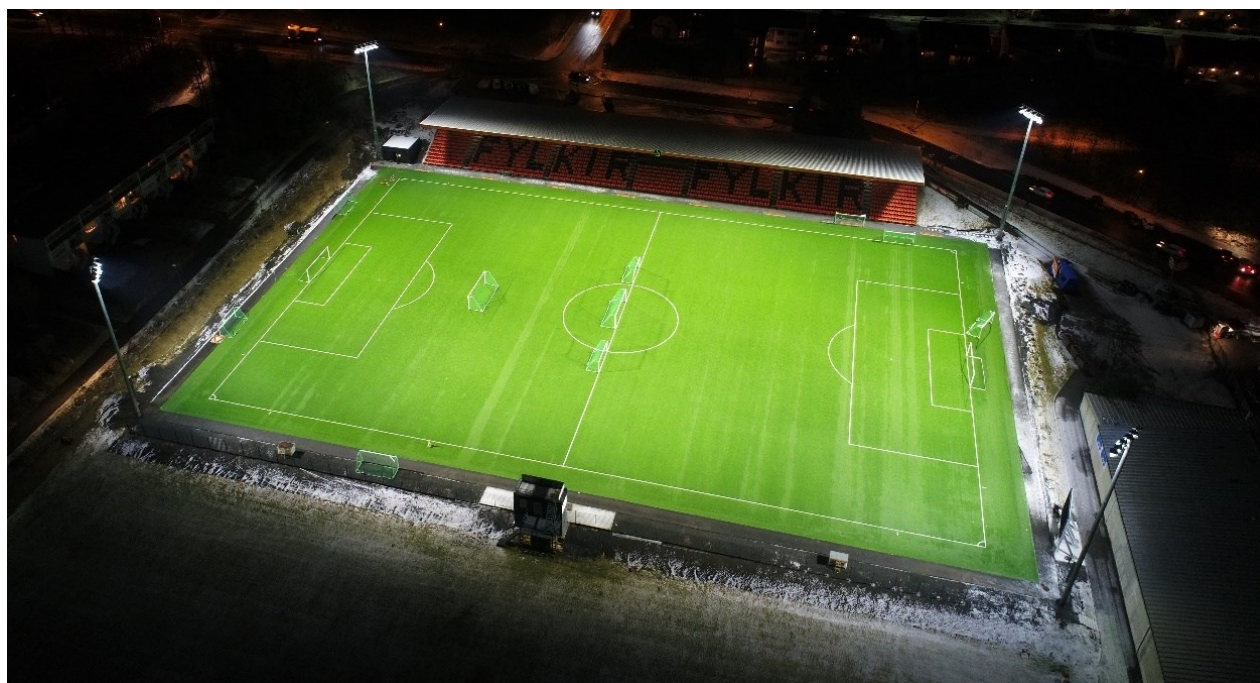
Figure 8: The Fylkir stadium – Lautin, Reykjavik; a winter photo taken after laying of the artificial turf with heating system in 2018. No snow is seen on the surface of the pitch compared to the surroundings.
