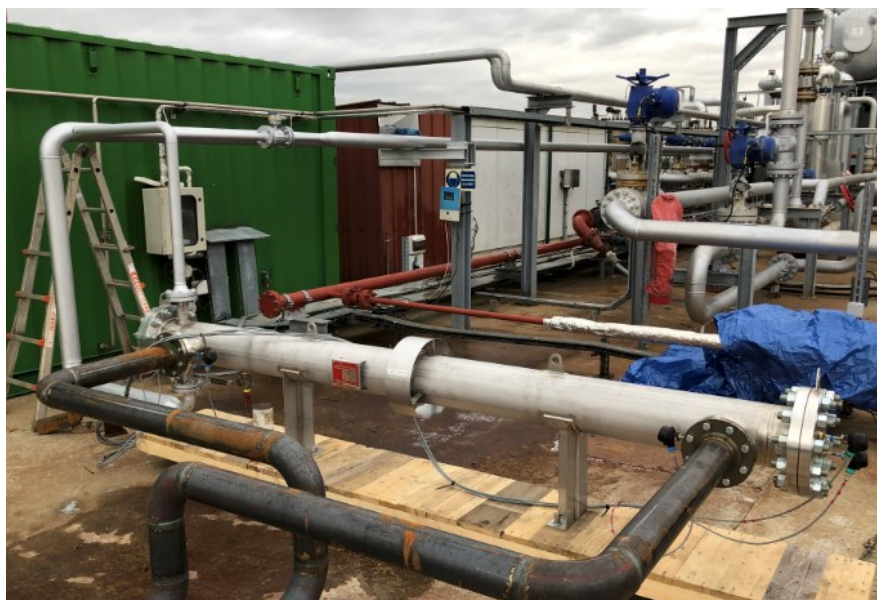
Figure 1: Test heat exchanger installed in Soultz power plant in 2019 (Ravier et al., 2019; Seibel et al., 2020).
