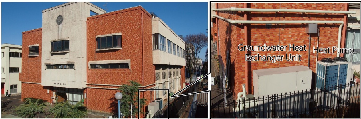
Figure 2: (Left) Heating/cooling experiment site. (Right) Enlarged image of the groundwater heat exchanger unit and the heat pump.
