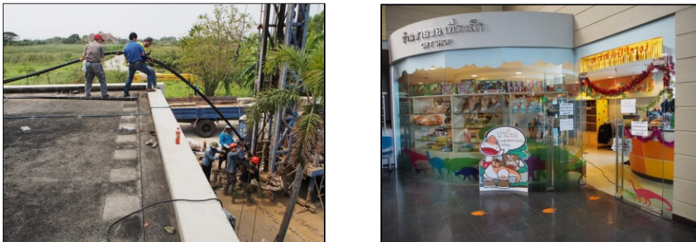
Figure 4. Installation of ground heat exchangers in Geological Museum, Department of Mineral Resources of Thailand
