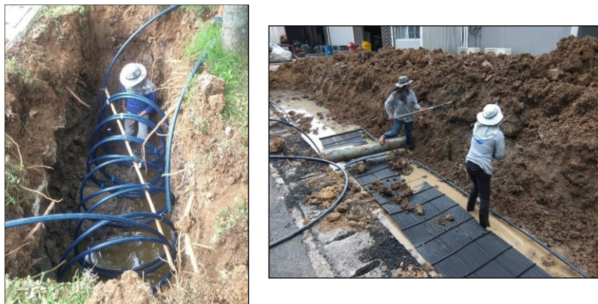
Figure 2. Installation of horizontal ground heat exchangers in Saraburi campus, Chulalongkorn University, Thailand.
