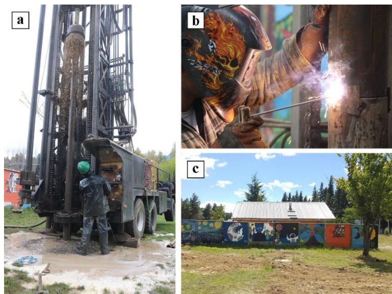
Figure 10: Boreholes drilling. a) Drill extracting ground water while drilling. b) Driller welding two steel pipes. c) Borehole final state.
