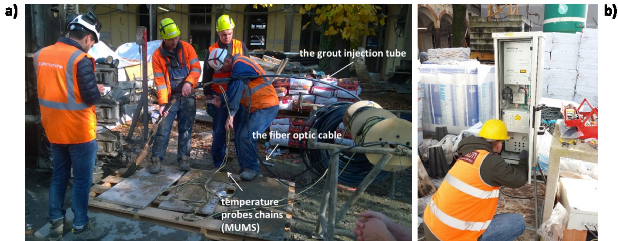
Figure 2: a) One phase of the installation procedure, with the hybrid fibre optic cable clamped to a rigid shaft and to the thermal sensor chains before the installation; b) the Distributed Temperature Sensing interrogator during the test.
