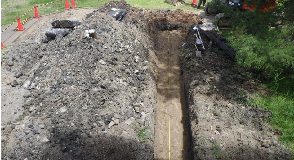
Figure 1: Schematic of field test site installed three Slinky-coil type horizontal ground heat exchanger under different ground surface coverage.
