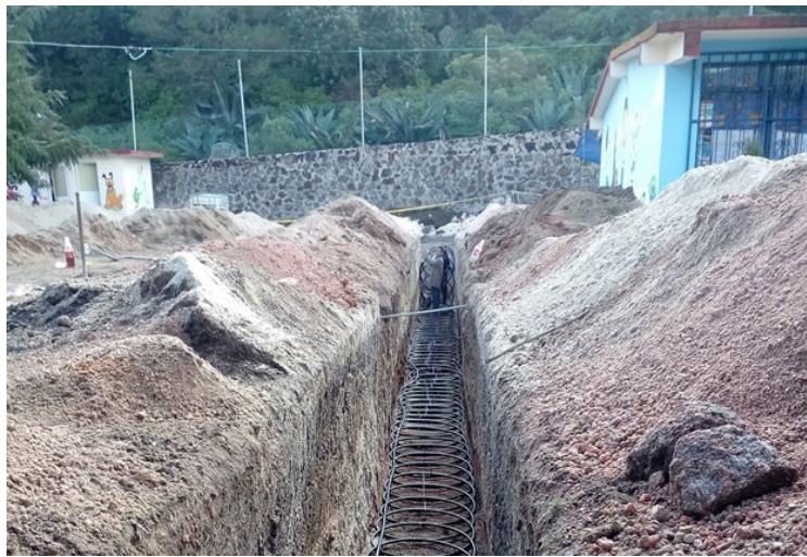
Figure 6: Horizontal ground loop to kindergarten building (INEEL, 2019)
