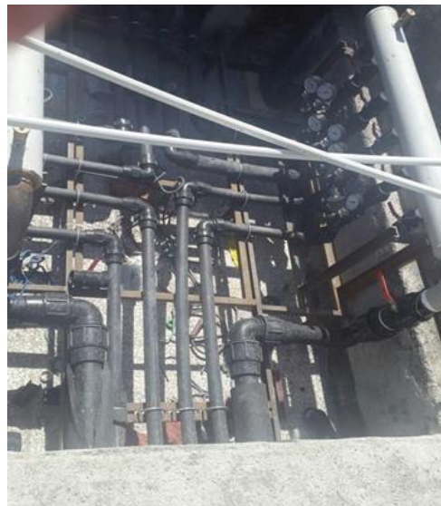
Fig4: Collector room for ground heat exchanger defined in Fig3 with thermometers and barometers on every circuit
