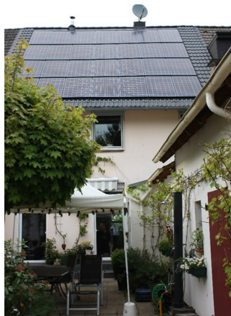
Figure 10: Family residence in Duisburg with a PV system to produce electricity for the household and the heat pump, EnergieAgentur.NRW (2017)
