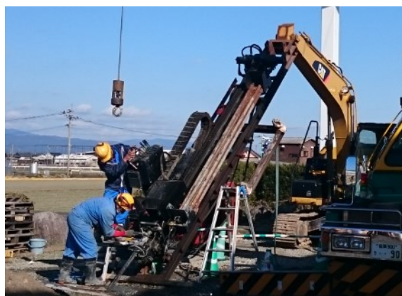
Figure 1: HDD equipment used for the horizontal GHE in Saga City, Japan
