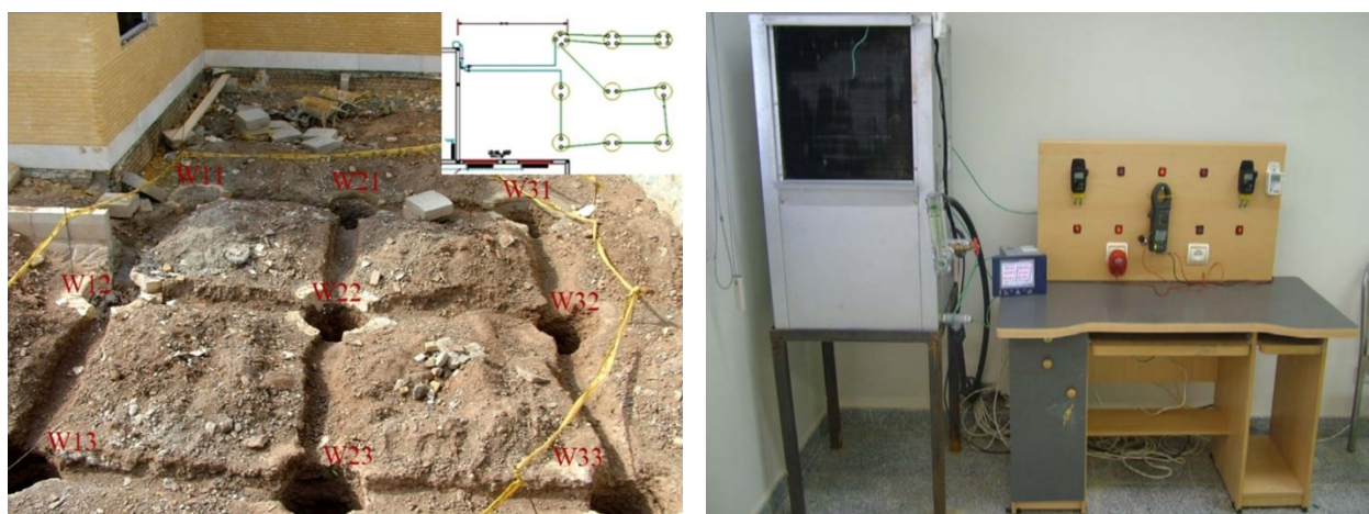
Figure 2: GSHP system which is installed in Taleghan, Iran. Drilled wells and schematic of the installed pipelines (left) and Heat Pump controlling devices and sensors (right).
