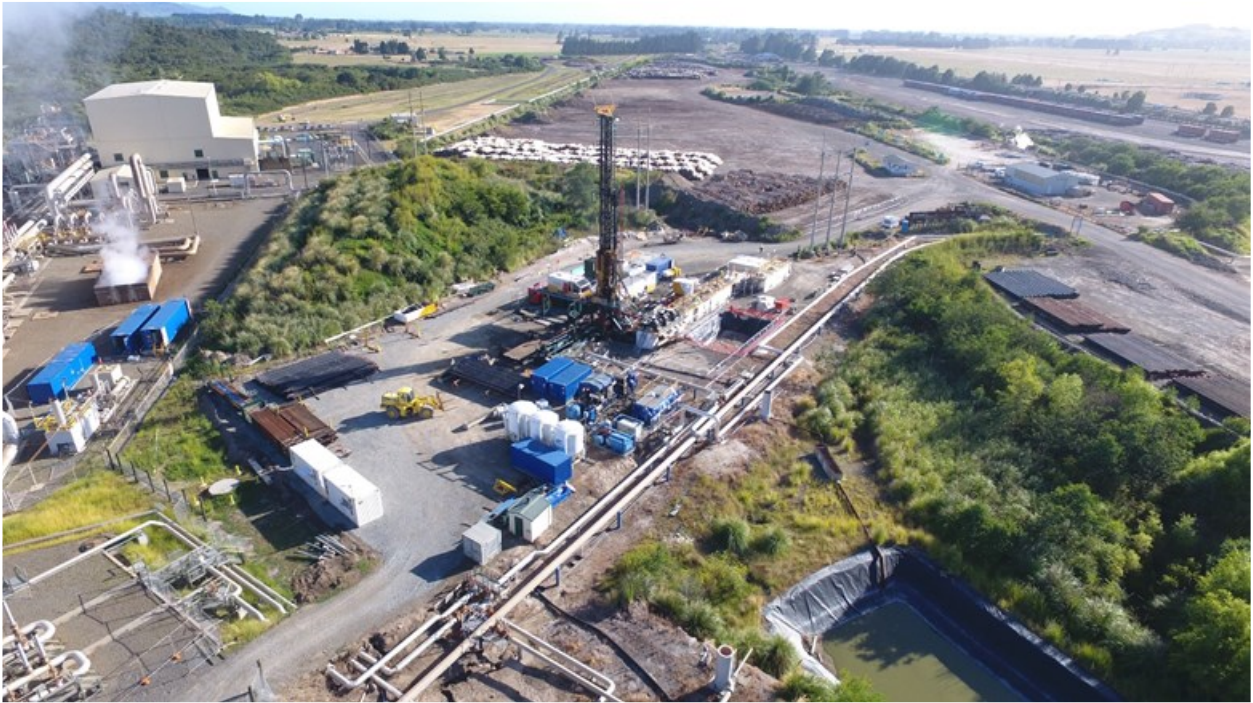
Figure 4. KA47 well casing repair on a tight well pad using Webber’s Nova-1 rig.
