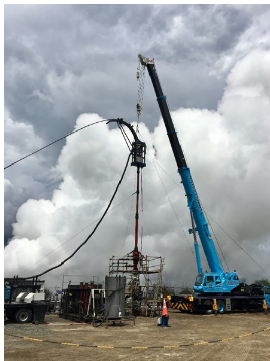
Figure 5. KA27 “live” clean-out using Western Energy’s coiled-tubing unit (CTU).
