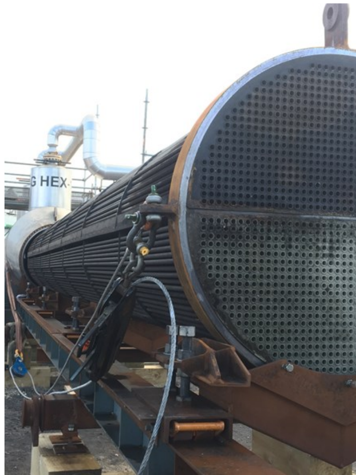
Figure 6. Tube bundle from one of the Clean Steam Plant heat exchangers during a recent routine maintenance and inspection. The fully redundant plant ensures clean steam supply was uninterrupted during this maintenance activity.
