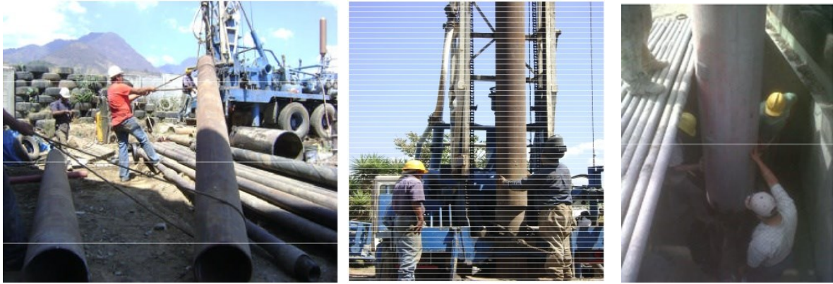
Figure 5: Setting the 14 inches casing in SM-2 Geothermal Well.
