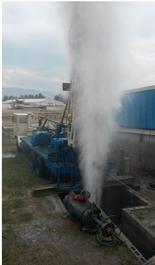
Figure 7: well SM-2 Flowing after setting up Casing.
