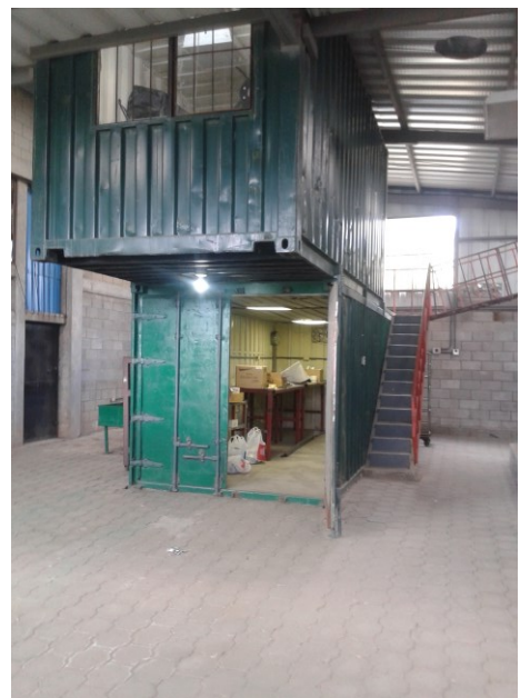
Figure 17: Converted Refrigerated Shipping Container into the Dehydration Tunnel. Regular shipping containers converted into the vegetable cutting and preparation area and lab.
