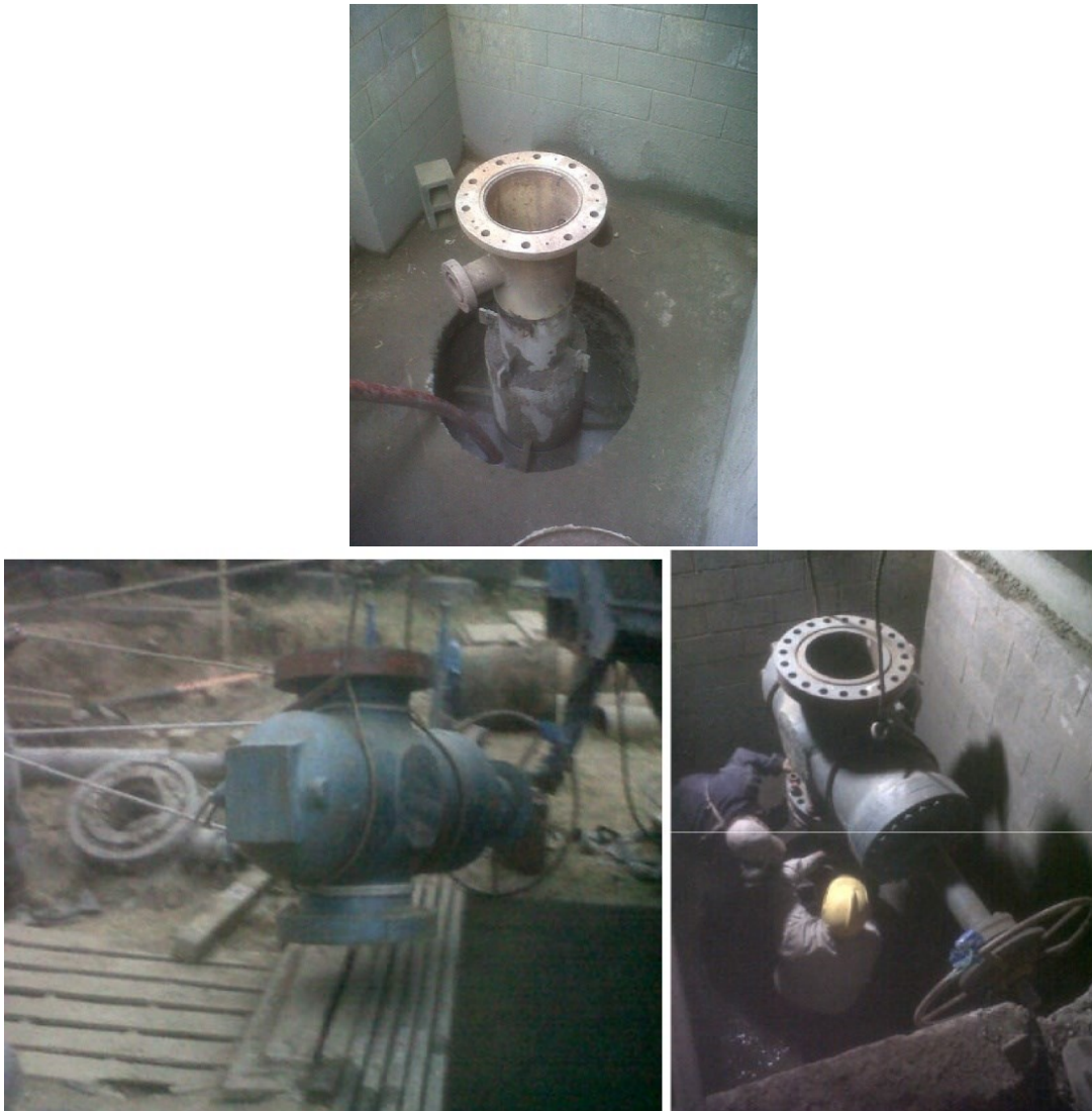
Figure 6: Cementing the well head and installation of main Valve in well SM-2
