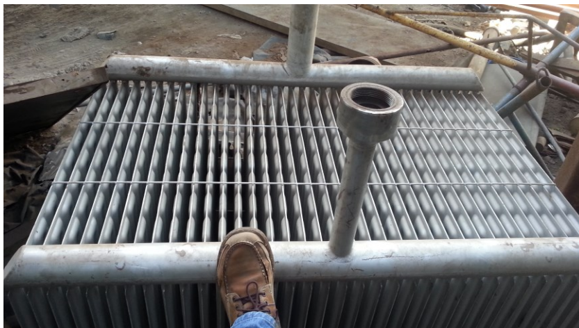
Figure 15: Off the shelf air conditioner/heat exchanger used in the refrigeration industry made of stainless steel and installed inside the water stack where the hot water of the well flows.
