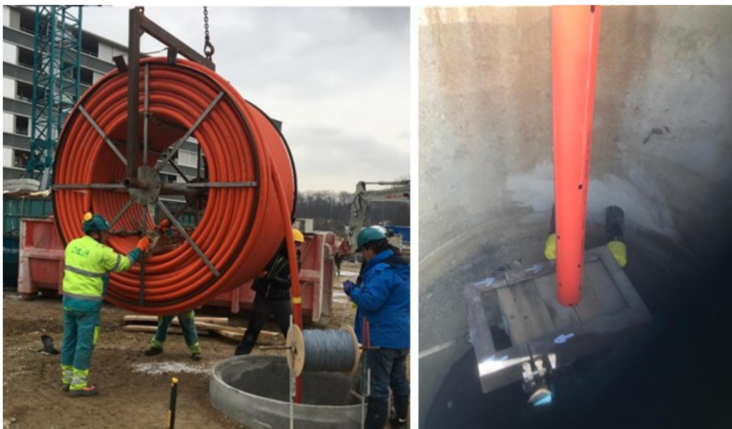
Figure 3: Installation of spoolable tubing (photos provided by V Cardon – Orllati, 2020 for a project in Switzerland)
