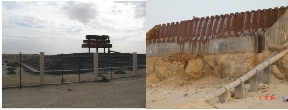
Figure 3: The water cooling system in cascade (case of Kebili area).
