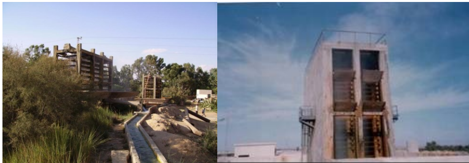
Figure 4: The water cooling system by atmospheric tower (Elhamma and Kebili areas).
