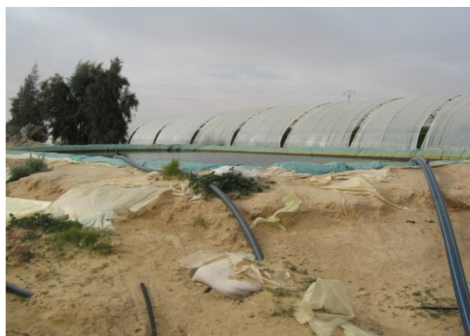
Figure 11: Type of small ponds with plastic linings to store the return water.
