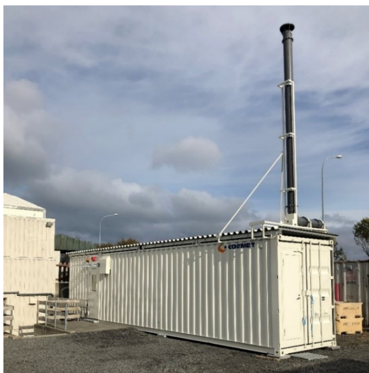
Figure 1: The corrosion laboratory constructed in a modified 40-foot high-cube container by Cormet Oy, Finland, shipped to Iceland, and installed at the campus of the University of Iceland.
