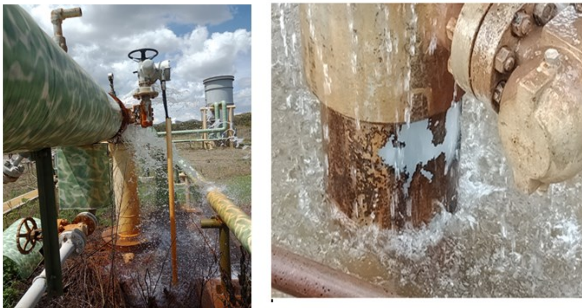
Figure 2: Corroded reinjection well OW-902A in Olkaria Domes field
