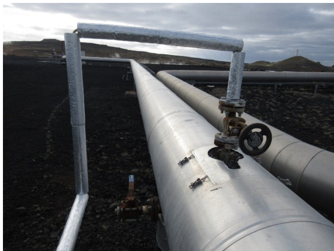
Figure 1: Sampling point used as a steam source.
