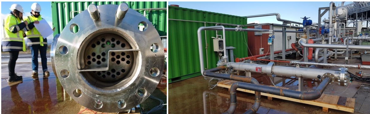
Figure 4: Prototype heat exchanger inspection (left) and final installation (right) [source és]
