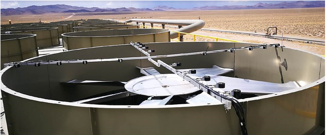
Figure 8: Continuous air flowrate measurement device
