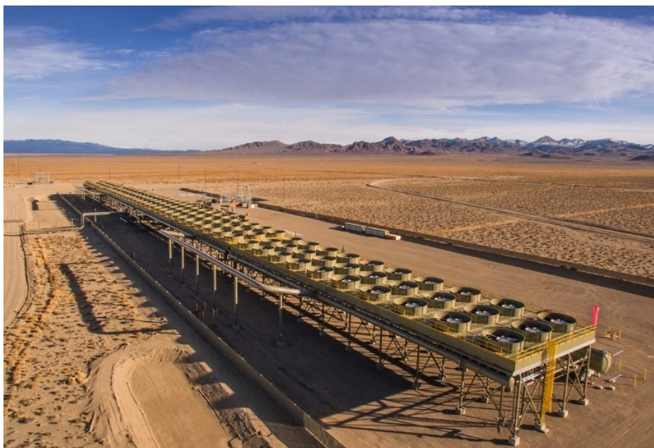
Figure 1: Don A Campbell Air Cooled Condenser
