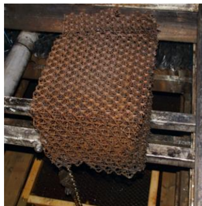
Figure 14: Inspection of STAR X20 3D filling media after about 1 year of operation.
