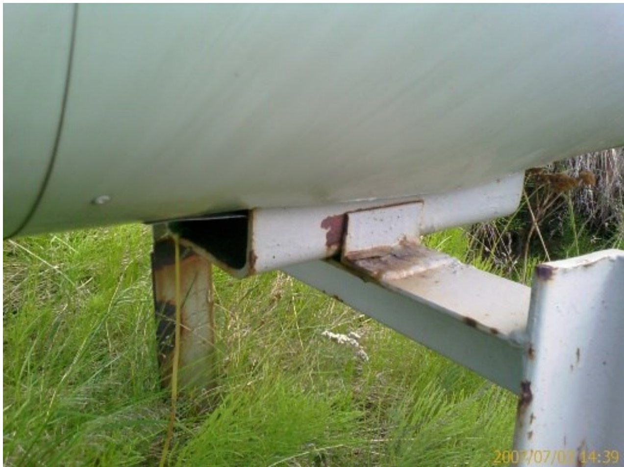
Figure 11: Support with only horizontal movement
