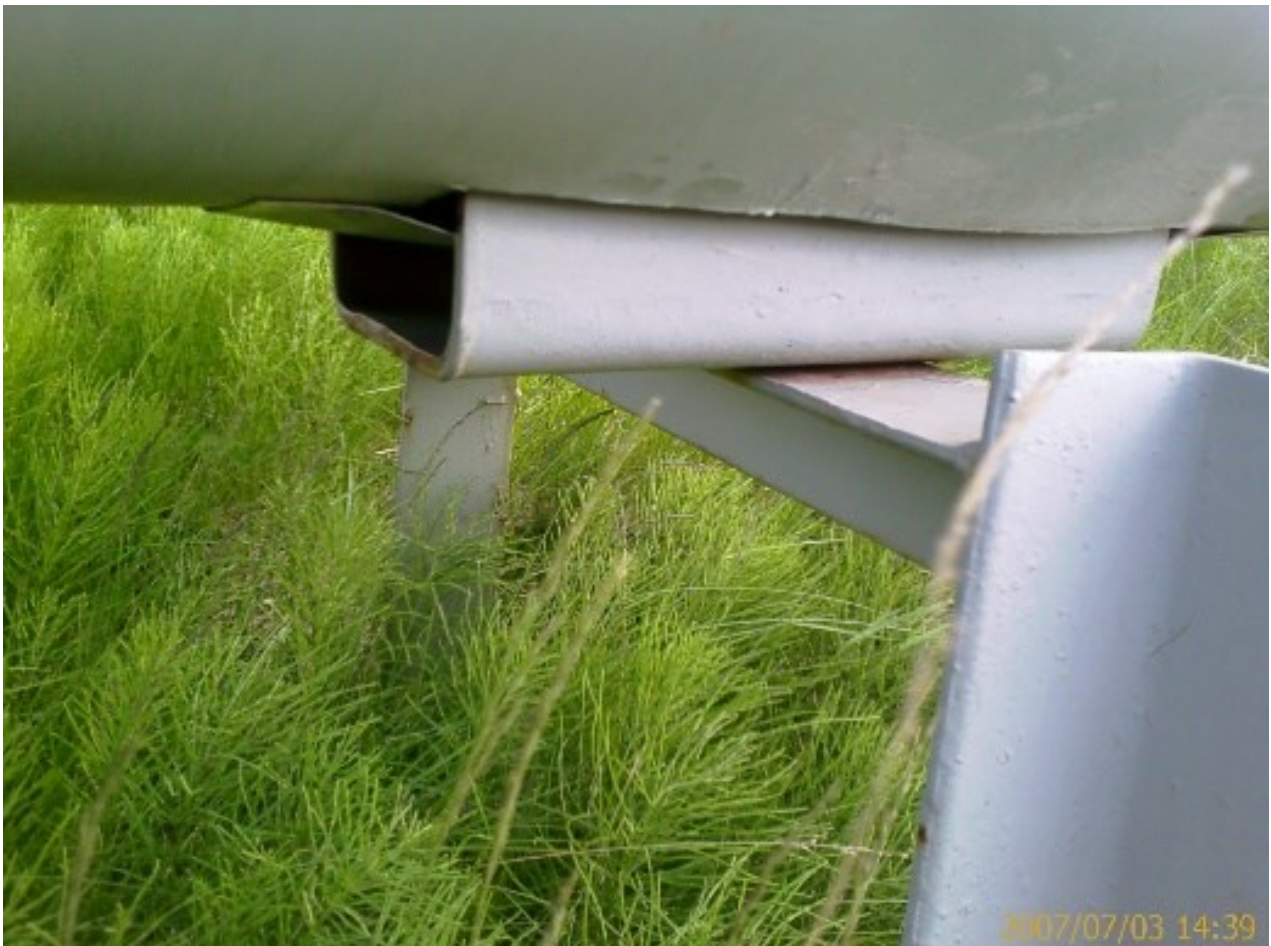
Figure 10: Support with horizontal & vertical movement
