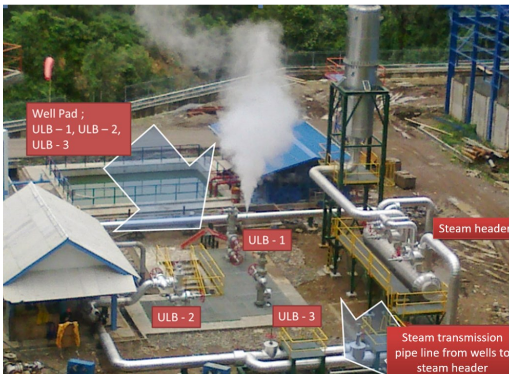
Figure 9: Challenge maintenance ability of ULB exploration wells due surrounded by main steam transmission line.
