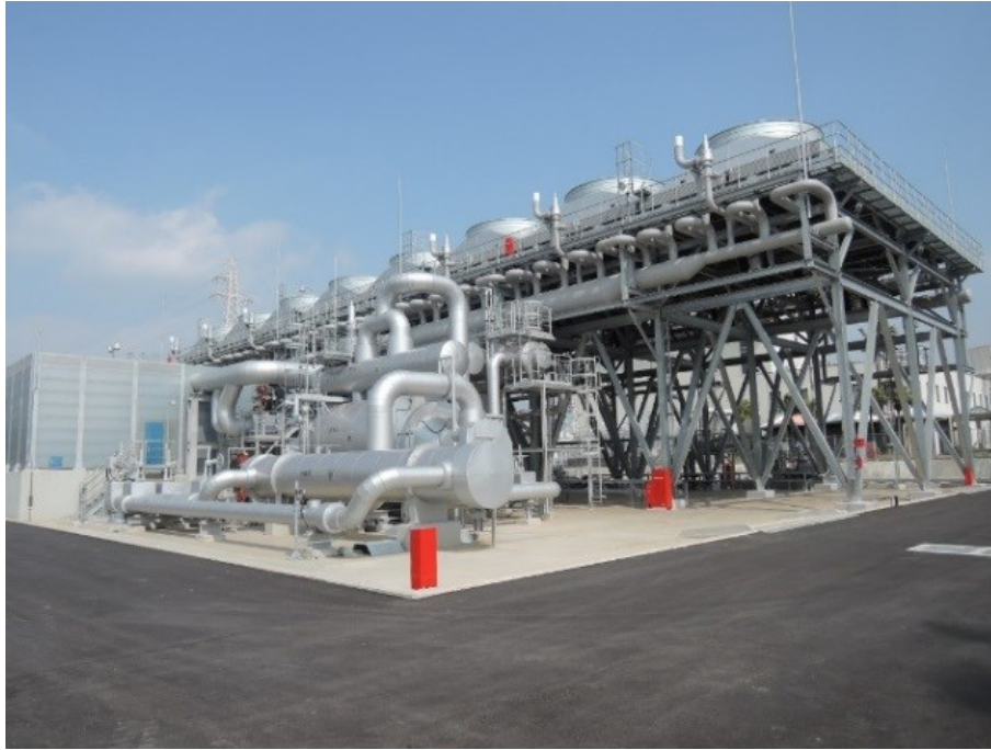
Figure 9: Heat exchangers.
