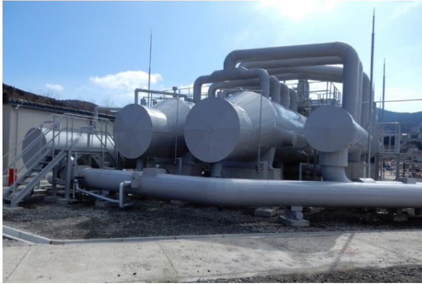
Figure 4: Preheater, evaporators and super-heater.
