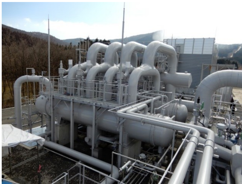
Figure 5: Water cooled condensers and recuperator.
