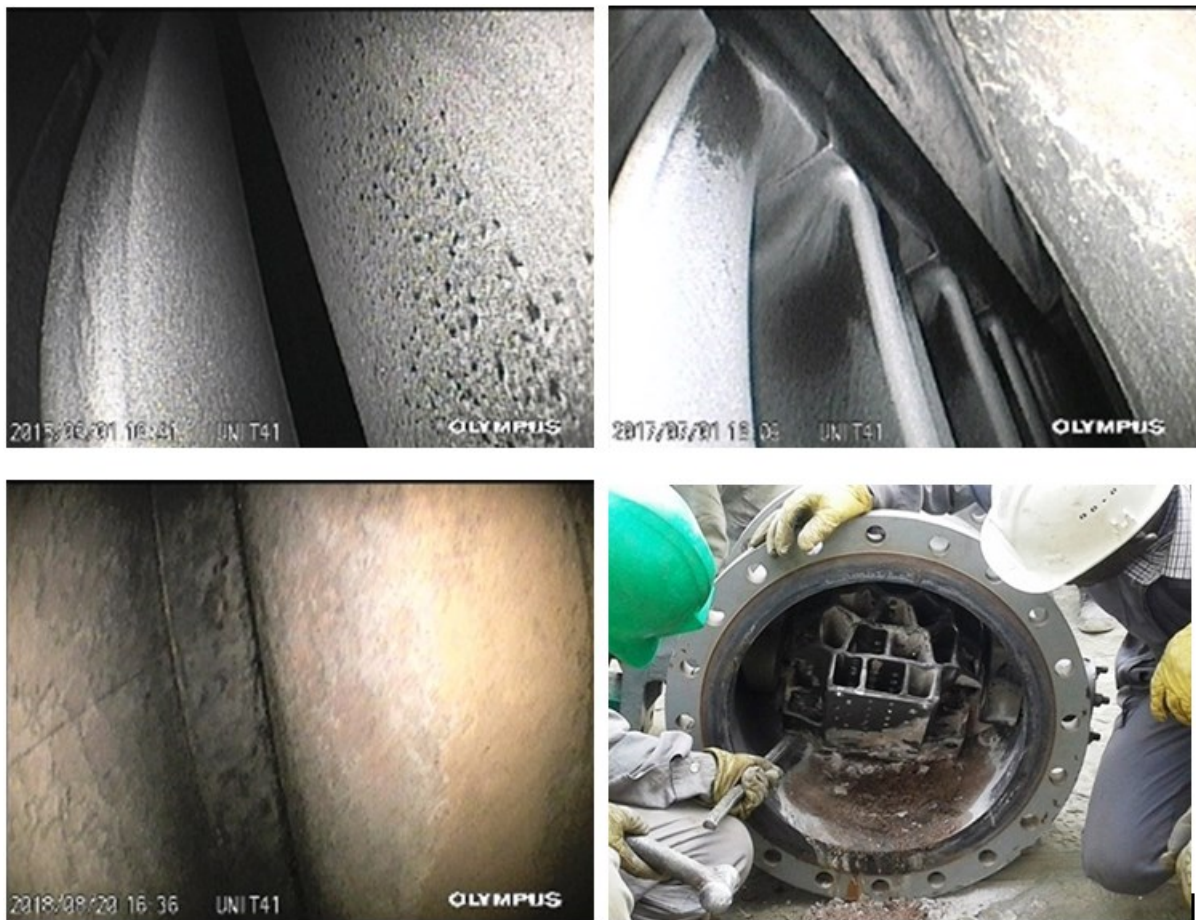
Figure 9: Olkaria IV turbine blades and scaling management in Olkaria IAU pressure letdown station.
