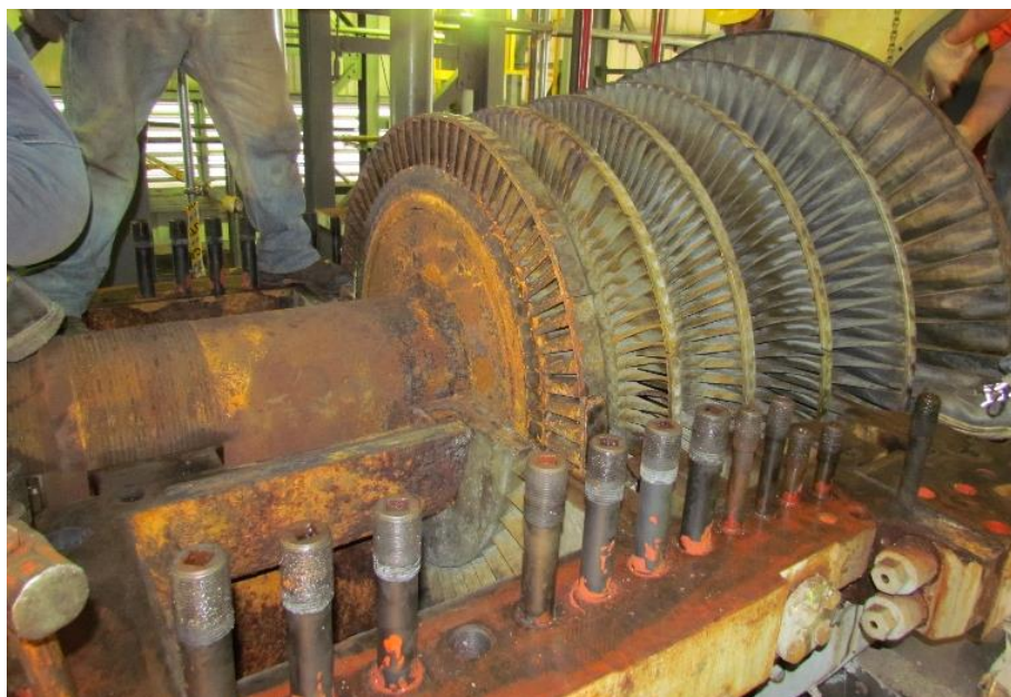
Figure 4. Typical appearance of a single flow turbine after lifting top casing
