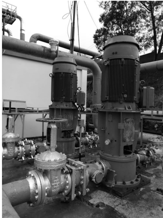
Figure 4: The Illated Centrifugal Vertical Pump
