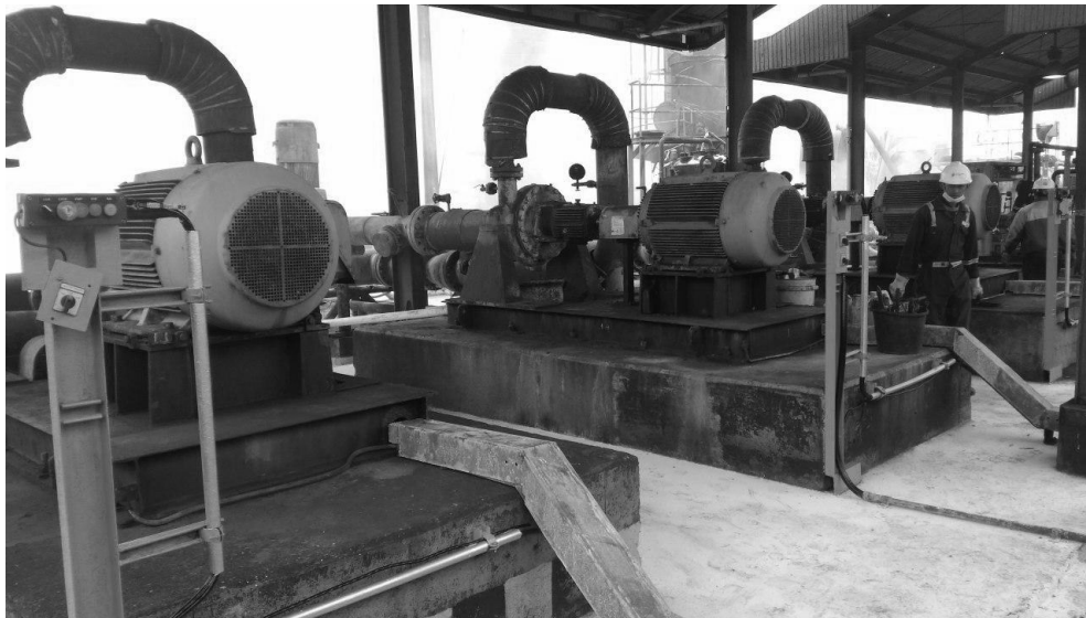
Figure 6: The Installed Centrifugal Horizontal Pump
