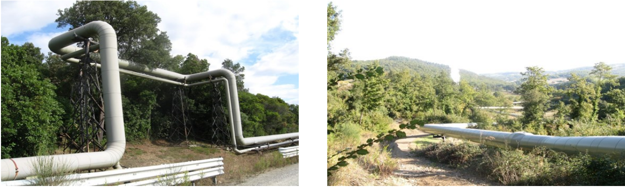
Figure 3: U-shaped and zigzag expansion loops.
