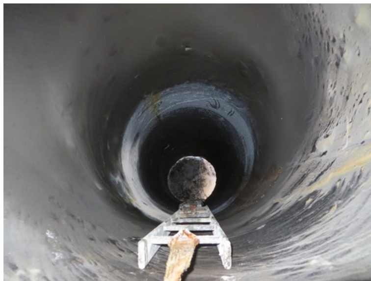
Figure 8: Barometric outlet pipe from LP-separator after 5 months.
