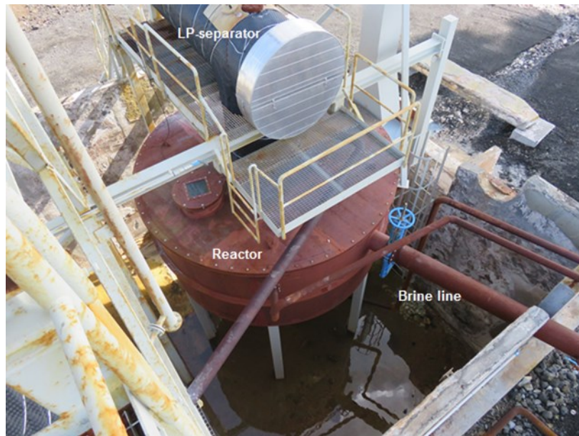
Figure 5: Reactor and LP separator
