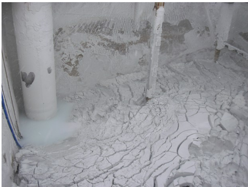
Figure 1: Silica sludge in brine collection basin after 56 days.
