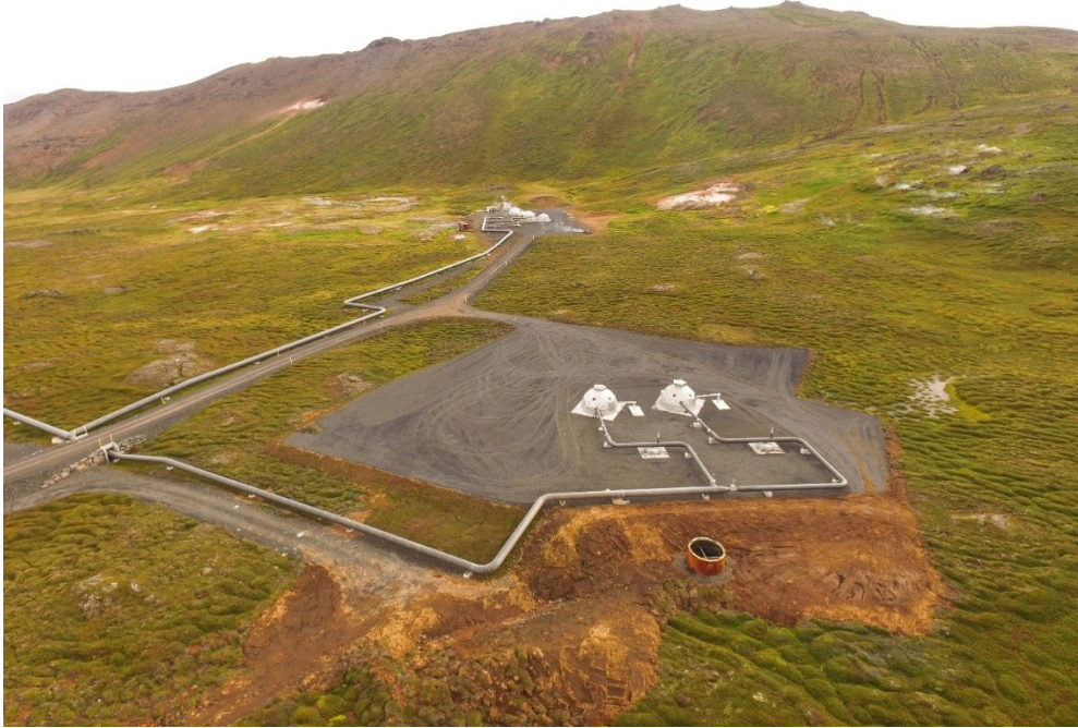
Figure 6: Drilling area C with wells ThG-12 and 16 in the foreground and wells ThG-03, 06 and 07 in the background. The joint silencer for ThG-12 and 16 can be seen at the edge of the drilling area.
