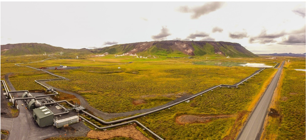
Figure 7: Overview of the steam field. The geothermal fluid is collected from the drilling areas and piped to the steam separators (bottom left). The steam pipelines continue to the powerhouse (left) and the separated water is sent to reinjection (bottom).
