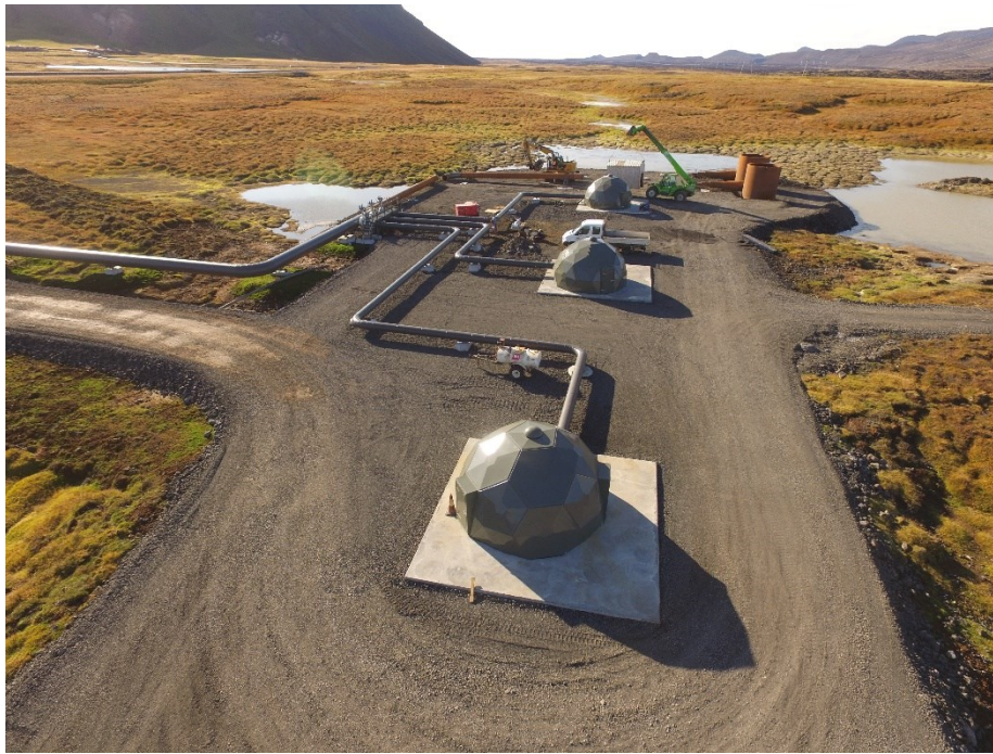
Figure 9: Reinjection wells, the emergency discharge is being installed in the background.
