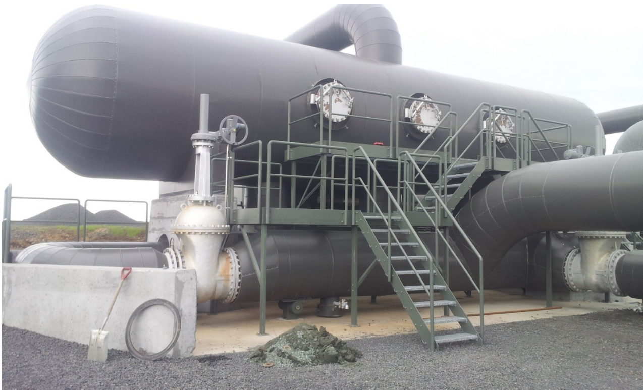
Figure 8: Steam separator.
