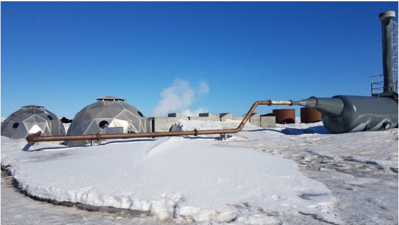
Figure 3: Apparatus used for the first-phase of the experiment in Beistareykir, Iceland. The pipeline can be seen connecting the geothermal well ÞG-18 and the steam separator.
